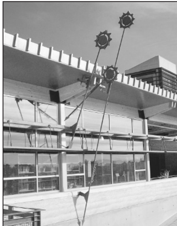
Roof eaves at the Springs Preserve's Desert Living Center restrict summer sunlight from hitting south-facing walls, but allow the benefits of light and heat in the winter, when the angle of the sun is lower. The ornamental arrows depict the angle of sun at summer and winter solstice.
