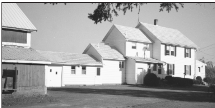
A connecting barn complex in Hadley, Massachusetts. Photograph by Richard Wilkie.
